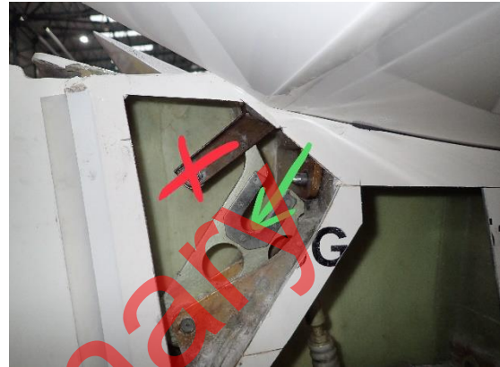
Disconnected elevator control
